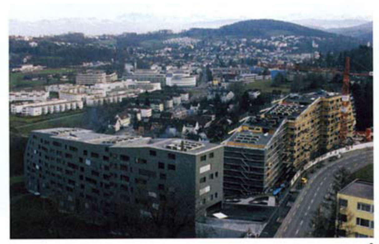
1 Generous balconies animate the stern slate-clad facades. 2 Edge of town context.
