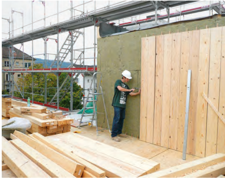
A worker installs the horizontal pegs that connect the posts into a continuous wall.
