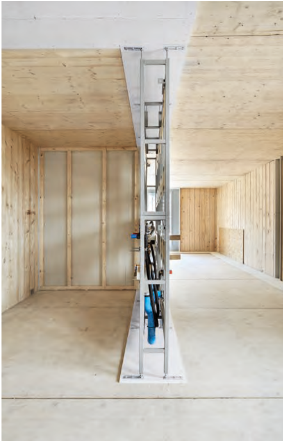
Non-load-bearing walls within the building consist of wood and metal elements depending on the service systems running through them.
