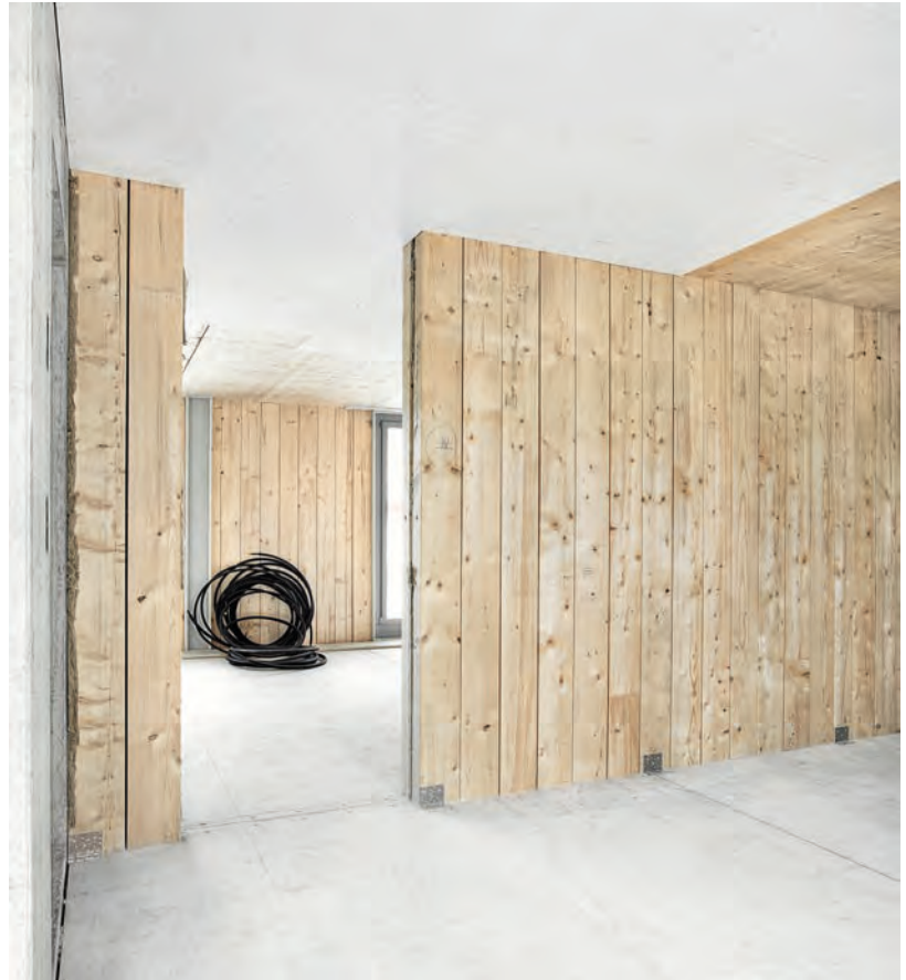
Wall prior to application of gypsum board. Notice the metal brackets used to stabilize and connect sections of the wall to the floor beneath.
