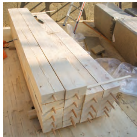
The 'Top Wall' system before and during construction. The pegs are already inserted and the posts are about to be installed.
