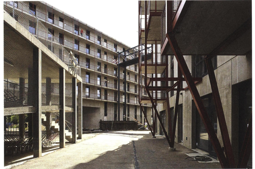
PROJECT: ZWICKY AREAL, SECTION E ARCHITECT: SCHNEIDER STUDER PRIMAS ARCHITEKTEN LOCATION & YEAR: DÜBENDORF (ZH), 2009–2015 IMAGE: ANDREA HELBLING, ARAZEBRA, ZÜRICH
