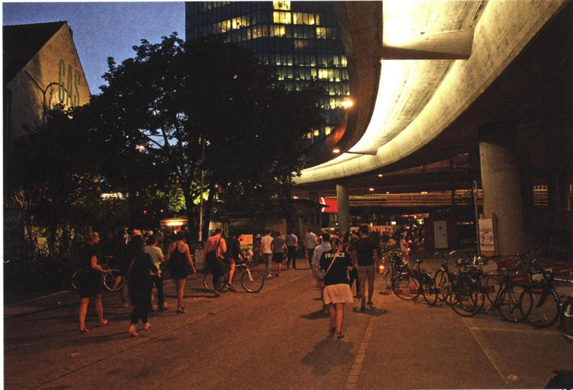
PROJECT: HARDBRÜCKE – GEROLDSTRASSE – LETTEN VIADUKT LOCATION: ZÜRICH (ZH) IMAGE: POOL ARCHITEKTEN
